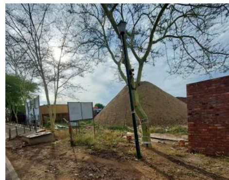
The insecure perimeter of the Maruleng Mall building site Image supplied
